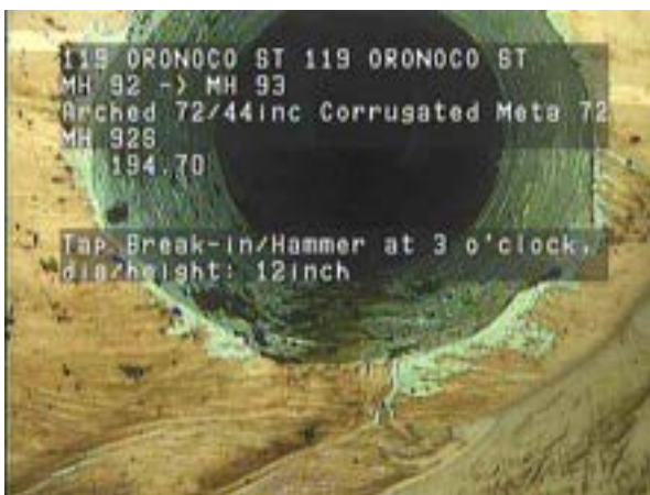
MH 92S_c02d2b53-7e83-4915-8b29-dfc666e74a32_20241217_15 1620_348.jpg, 00:09:00, 194.70ft Tap Break-in/Hammer at 3 o'clock, dia/height: 12inch
